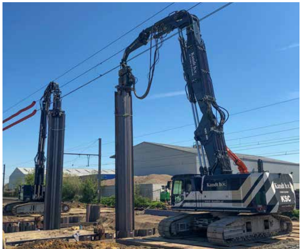
Installation by vibratory hammers with double clamping systems mounted on hydraulic rigs
