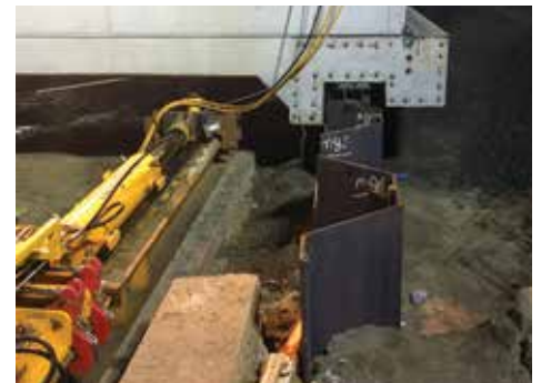
Pushing of the prefabricated bridge deck over sheet pile abutments
