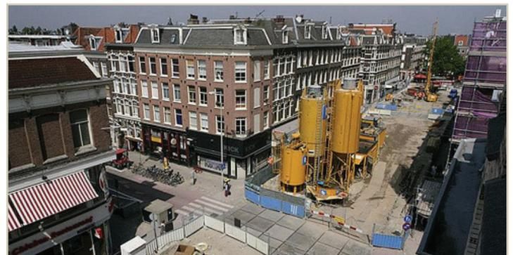
Figure 3.7. Fluid treatment plant, bentonite and cement silos at inner-city project North South Line Amsterdam, the Netherlands.
