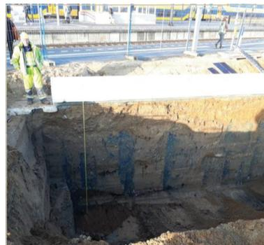
Figure 3.13. SoilMix wall excavated in vicinity of active railway, station Blerick, the Netherlands.
