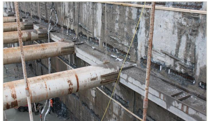
Figure 3.6. Connection with concrete deck and struts during excavation, project Garenmarkt, Leiden, the Netherlands.
