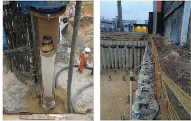
Figure 3.15. Secant pile wall, installation (left) and excavation (right), <https://www.vsf.nl/nl/funderingen/wanden/boorpalenwanden>.
