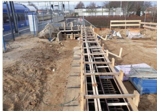
Figure 3.12. Capping beam on top of SoilMix wall in vicinity of active railway, station Blerick, the Netherlands.
