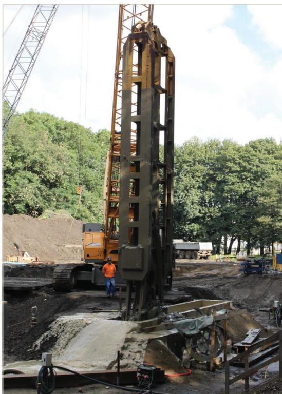
Figure 3.5. D-Wall grab with sled and elevated bentonite level, test site Noord Kasteel, Antwerp, Belgium.
