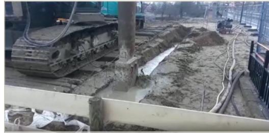
Figure 3.11. SoilMix wall in execution in vicinity of active railway, station Blerick, the Netherlands.
