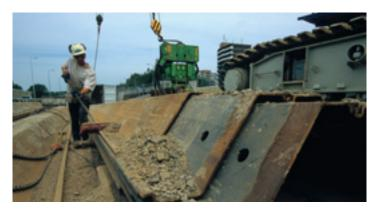
Steel sheet piles are very suitable for use in temporary constructions such as building pits, pipe trenches, dams, etc. Steel sheet piles can easily be removed and re-used.
