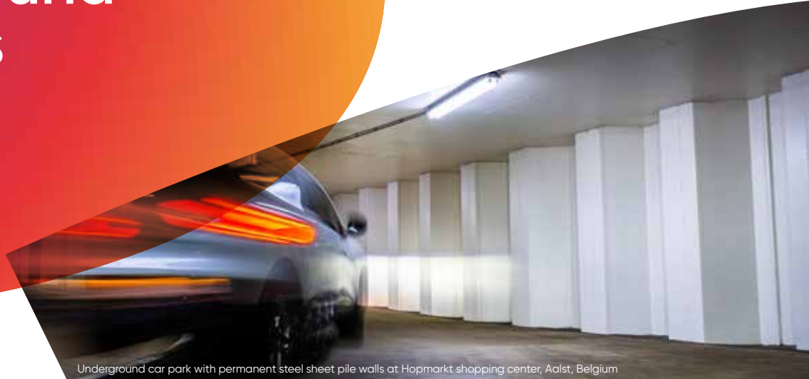
Underground car park with permanent steel sheet pile walls at Hopmarkt shopping center, Aalst, Belgium
