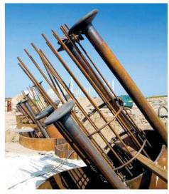
Example of a steel tube as anchoring element
