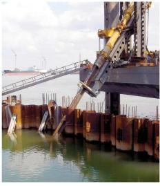
Installation of MV piles
