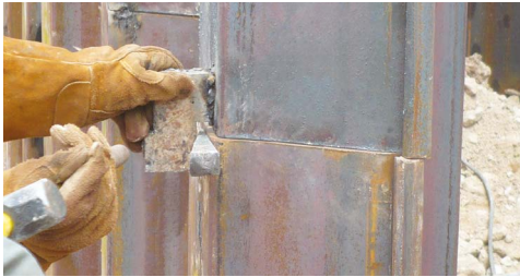
Aligning the interlock position to allow sliding of profiles after welding
