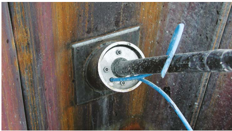
Watertight connection for a grouted anchor
