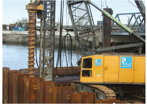
Pre-drilling for intermediary piles of a combined HZ ® -M wall
