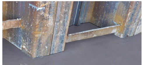
Welded lash to fix the profile in the intended width
