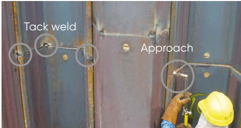
Example of a construction joint
