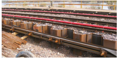
U-piles with waling along a railway line
