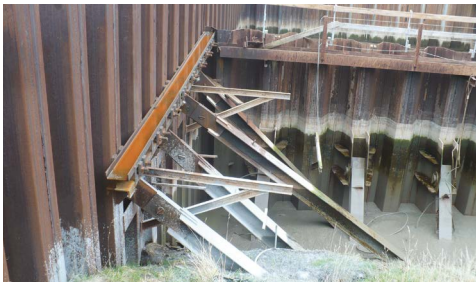
Inclined pile connection
