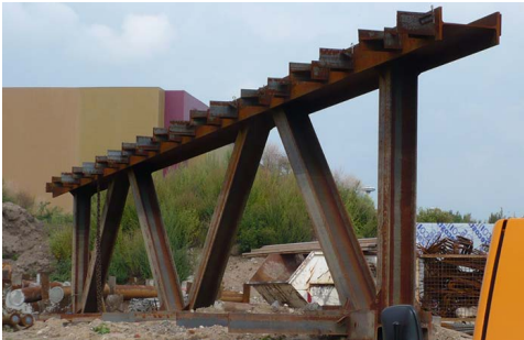
Special open guide, only holding the HZ®-M beams at the rear flanges
