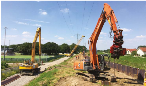
Excavator-mounted vibrator
