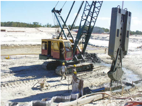
Example of a cut-off element
