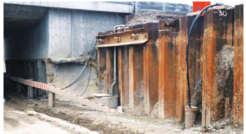
U-profile as waling for temporary piles
