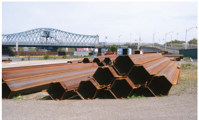
CAZ storage area
