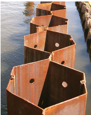
Completed CAZ box pile wall
