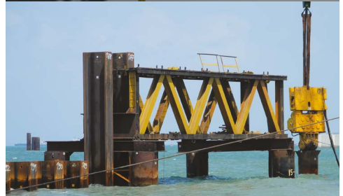
Guide frame with two levels for the HZ ® -M system
