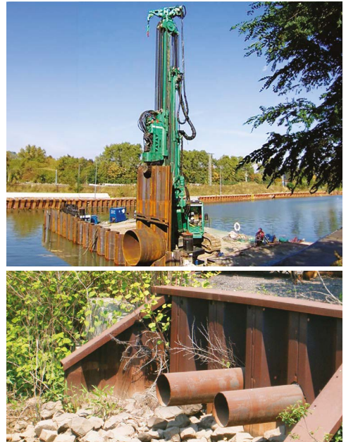
Examples of connections through sheet pile walls
