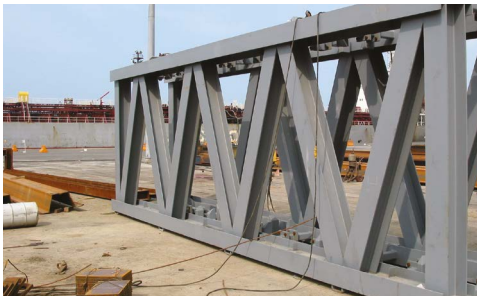
Example for a piling guide for a combined HZ ® -M wall, adaptable for different king pile sizes
