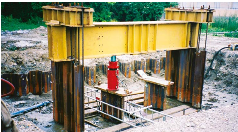
Example of a load test for a sheet pile wall
