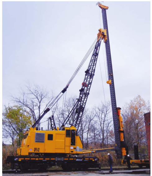
Rail-based pile driving rig.
