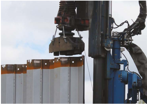
Driving cap under hammer
