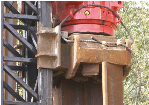
Driving cap placed on sheet pile wall
