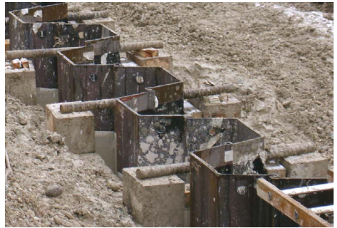
Holding equipment for sheet piles placed in a trench
