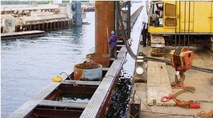
**A non-floating template.** The template rests on either auxiliary or already installed tubes of the combined wall. This type of template is more stable and can be used in more rough waters.
