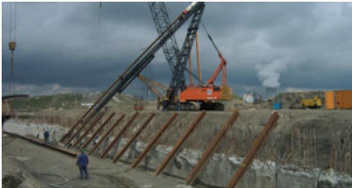
HP foundation piles can be charged with compression as well as tension. According to the application, the piles can be modified by enlarging the toe or by injecting grout during the installation process (MV piles). Injected piles can take very high tensile forces ( $\geq 500$  tons per pile).
