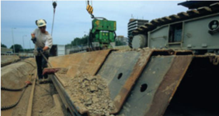
Steel sheet piles are very suitable for use in temporary constructions such as building pits, pipe trenches, dams, etc. Steel sheet piles can easily be removed and re-used.
