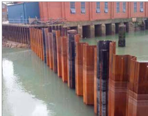
Fig. 12. Port of Shoreham. AMLoCor steel sheet pile wall.
