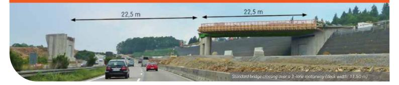
A case study, performed by the Karlsruhe Institute of Technology (KIT), assesses all associated costs and performance of a traditional concrete bridge versus a bridge whose abutments are constructed using steel sheet pile sections. This comparison is performed for a two-span superstructure with spans of 22,50 m and a superstructure width of 11,50 m accounting for a standard crossing of a national road over a 3-lane motorway with an average daily traffic (ADT) of 70'000 vehicles:
